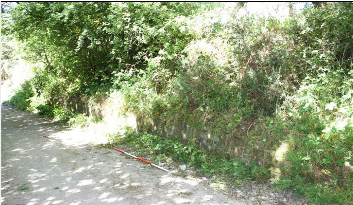
Plate 11: Wall continuation beyond area effected by proposed road scheme, looking north-west
