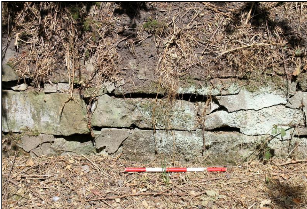
Plate 9: Section of wall that had been partially pointed with cement mortar
