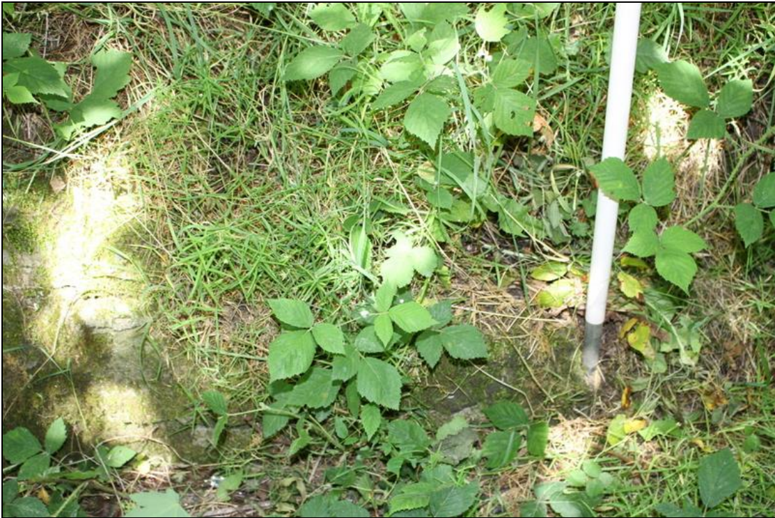
Plate 12: Apparent eastern terminus of retaining wall
