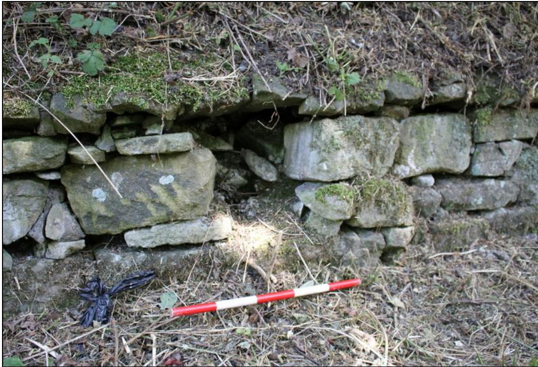
Plate 8: Exposed rubble wall core
