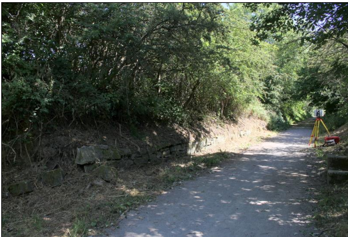
Plate 4: General view of the northern retaining wall, looking north-east
