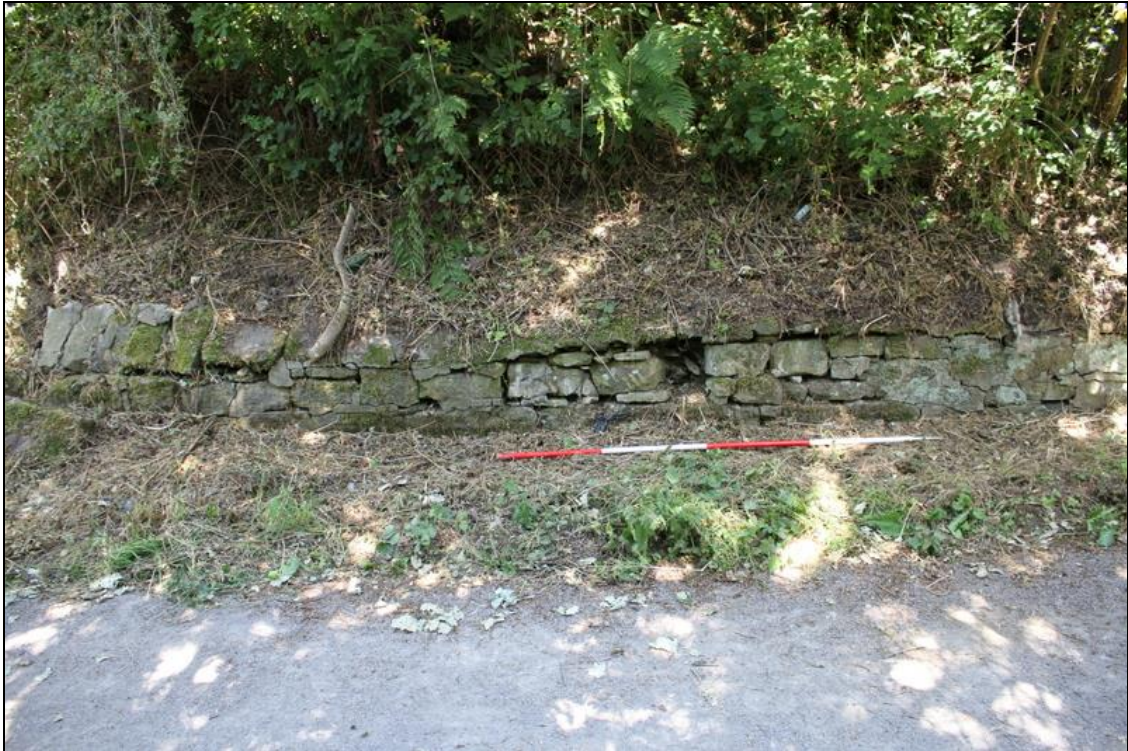
Plate 6: Detail of retaining wall construction
