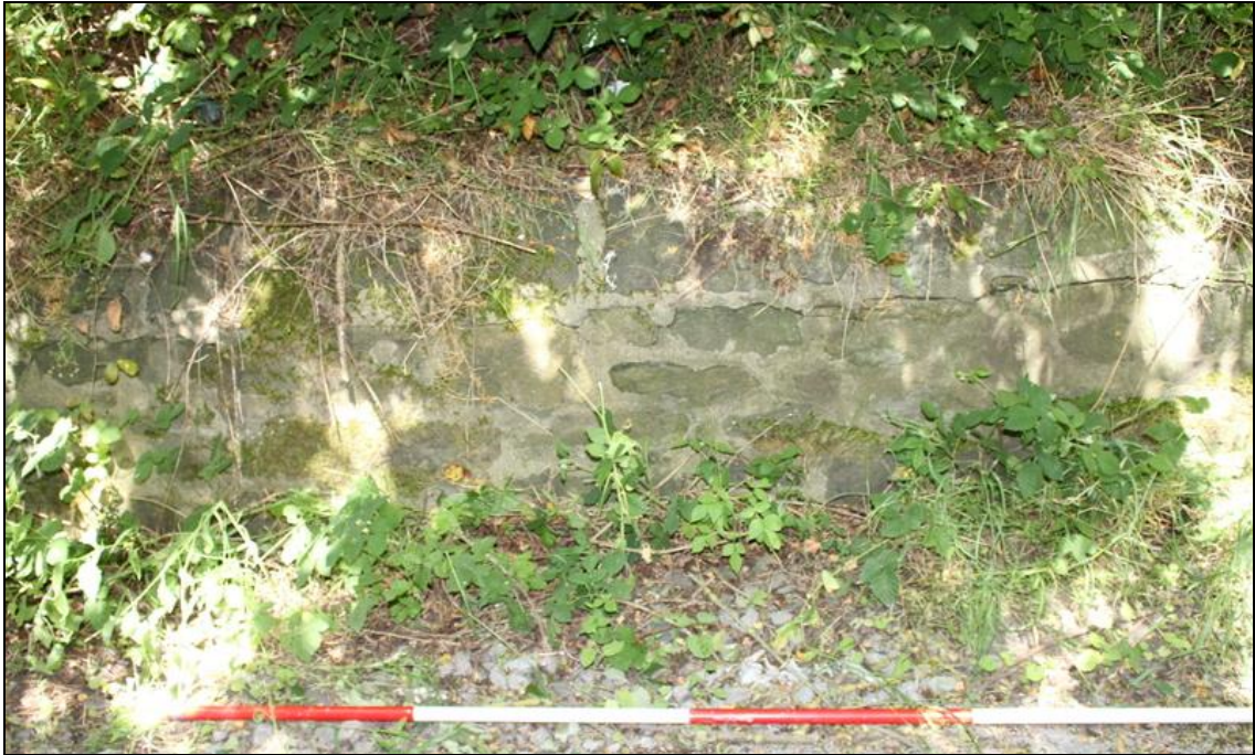
Plate 10: Struck cement pointing within section of wall to be retained
